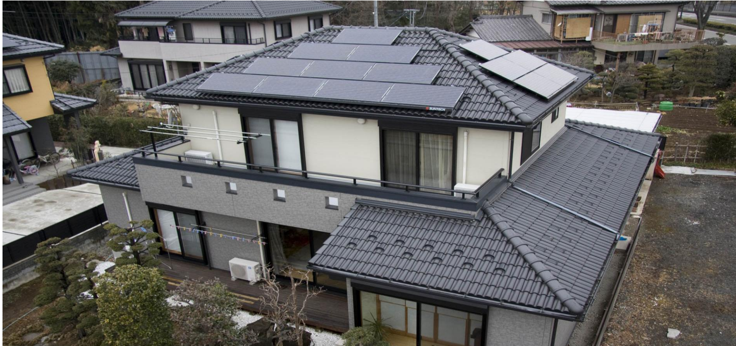
Residential Installation in Sapporo, Japan
